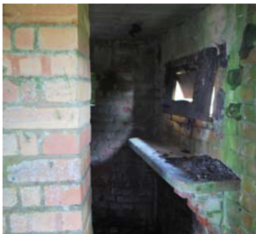
Fig 56 (below) Heavy machine gun loophole, metal shutter, firing shelf & anti-ricochet wall (Hazel Riley)
