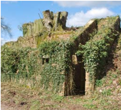
Fig 48 (above) Defended wall over the air raid shelter, fighter pen 229 (Hazel Riley)
